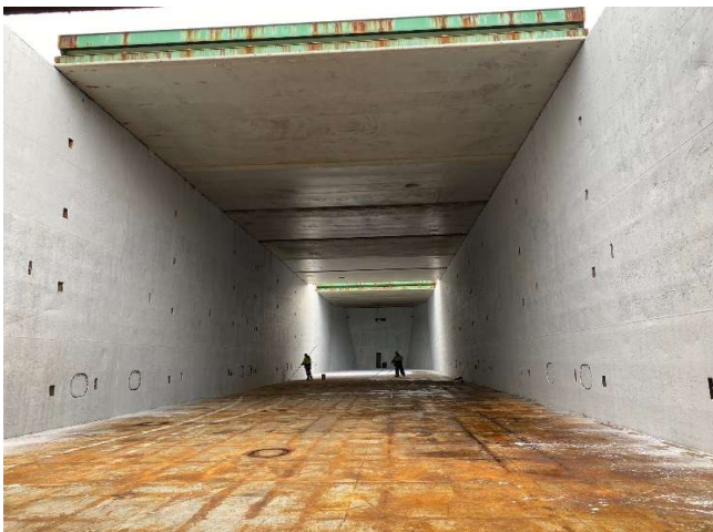
Hold looking Aft.
